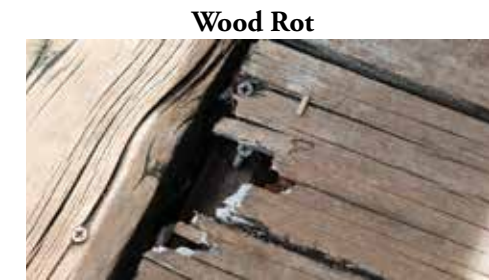
Shown Above: Ipe (Brazilian Walnut) Hardwood decking installed with face driven screws.
