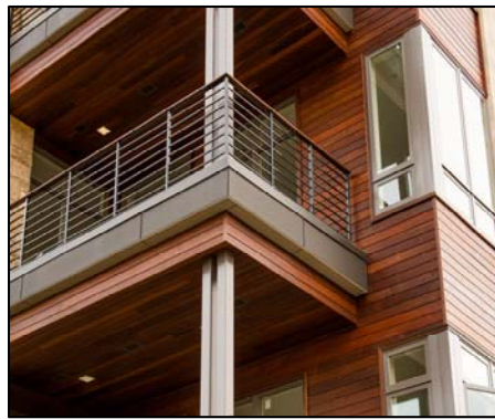
Rain Screen and Soffit
