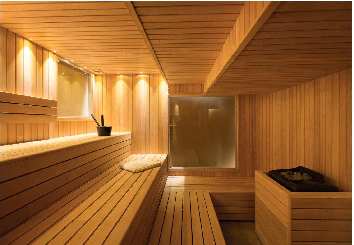
Walls: STP 1x4 alder, benches: SHP 5/4x4 alder. Spa sauna in Germany.
