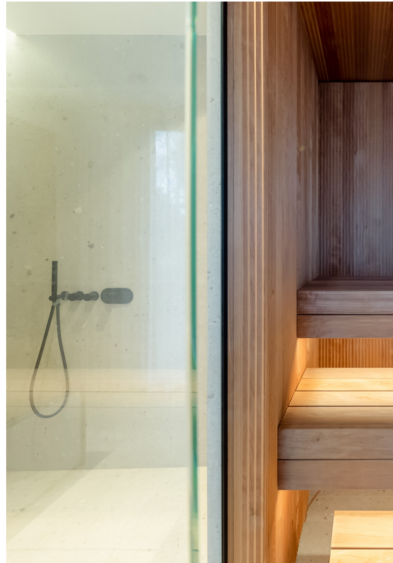
Walls and ceiling: Vire 1x3 thermo-aspens, bench: SHP 1x4 thermo-aspens. Private house, Estonia. Photo by Elvo Jakobson
